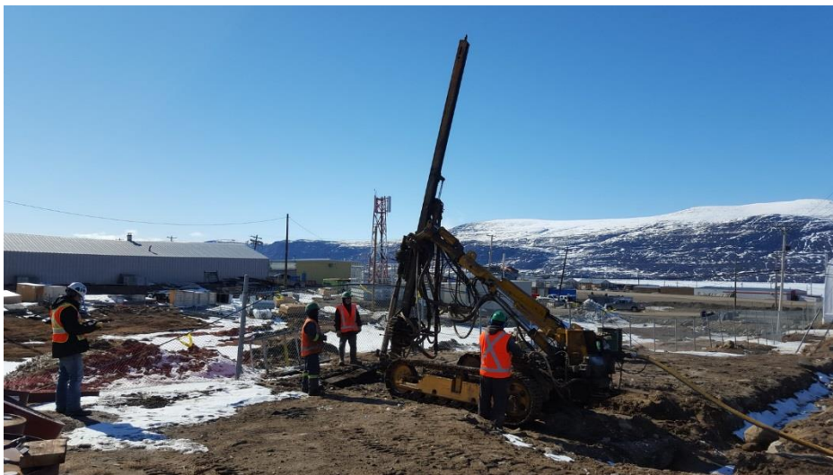
Pile installation at Pangnirtung power plant rebuild site
